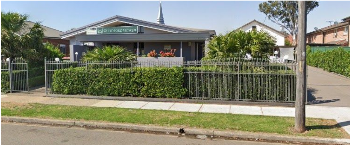
Figure 4: The subject site viewed from Mountford Avenue, showing main street frontage and existing buildings on the site 3
